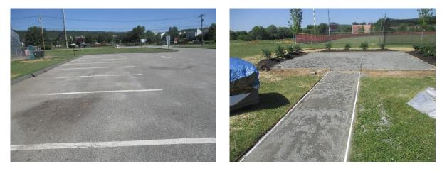
Parking spaces and the basketball court can be replaced with porous asphalt to infiltrate stormwater. A preliminary soil assessment suggests that more soil testing would be required before determining the soil's suitability for green infrastructure.
